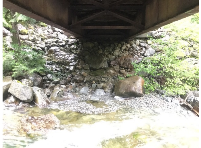
Left Bank Abutment when facing downstream
