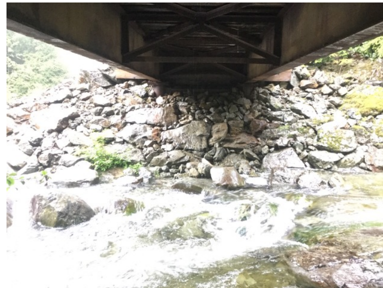
Right Bank Abutment when facing downstream
